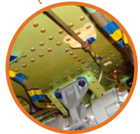
FLOOR FRAMING, PLATE/BOLT CONNECTIONS
